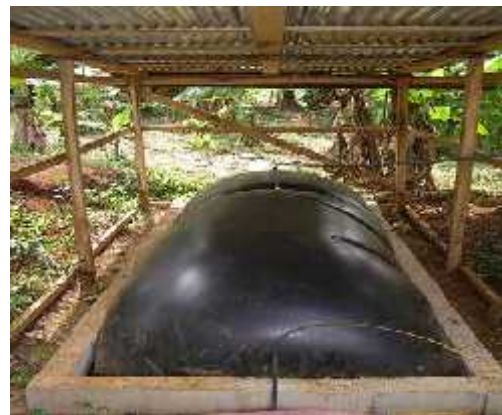
Gambar 3 Tipe Digester Baloon Plant
